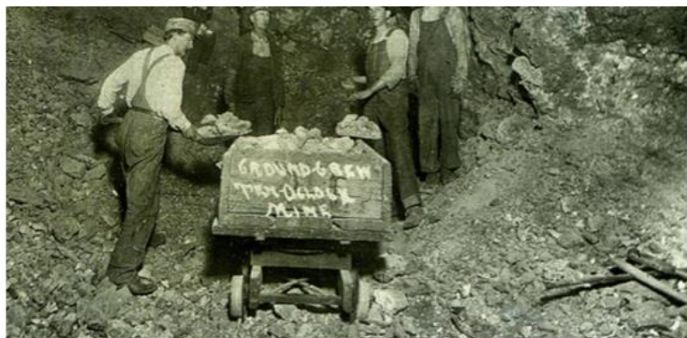
Lead & Zinc Mining in Joplin, MO - circa 1910. Two miners in the background examine the roof of the mine. From: Historic Joplin, "Men and Dust", http://www.historicjoplin.org/?tag=tri-state-mining-district
