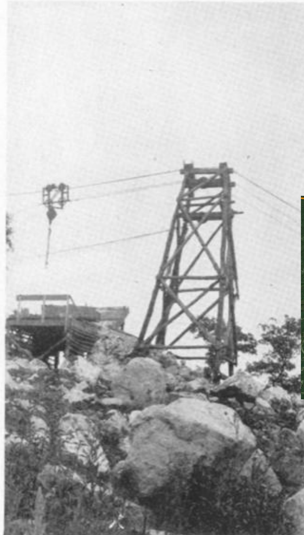
B. NEWELL MINE, NE \frac{1}{4} NE \frac{1}{4} SEC. 14, T. 41 N., R. 18 W. TRAVELING CRANE AND LOADING FACILITIES FOR TRUCKS.
